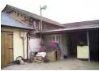
The old building before work.
