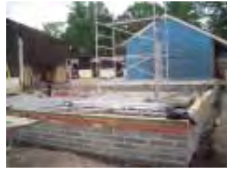
New foundations are put in
